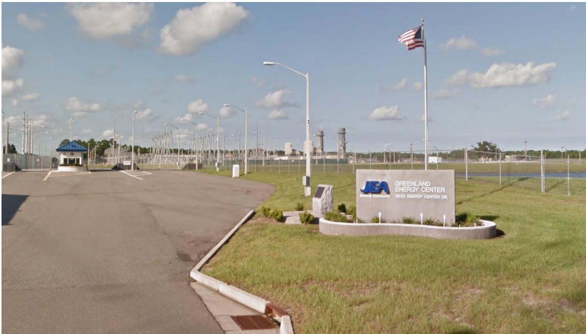
View of Property to the West
